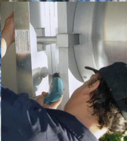
This GMP-1398 side-mounted drip pan is a cost-effective solution for rooftop grease spills. It is equipped with a disposable grease drape and a water drainage system that allows clean rainwater to flow without spilling grease onto a roof, and works well with or without a lid cover.
