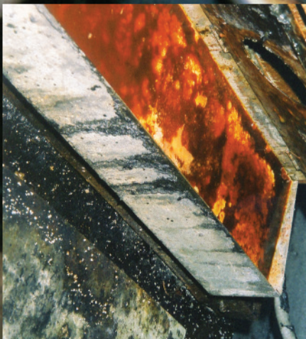
This collection box full of grease is about to overflow onto a roof.
