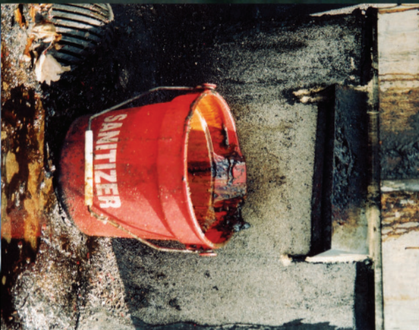
Roof damage caused by not maintaining or installing proper grease containment.
