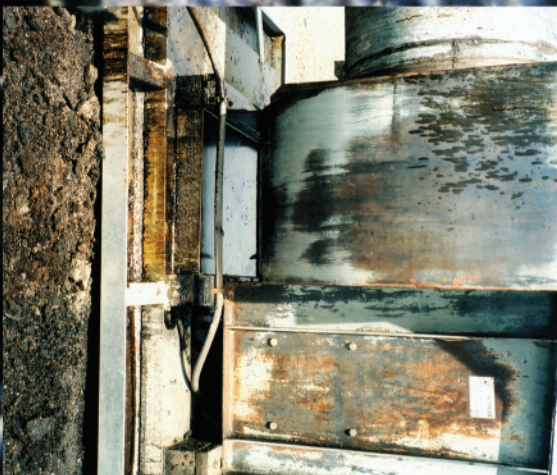
Roof damage caused by not maintaining or installing proper grease containment.
